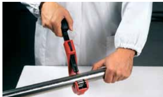
Figure 25 - Cutting the pipe to length
